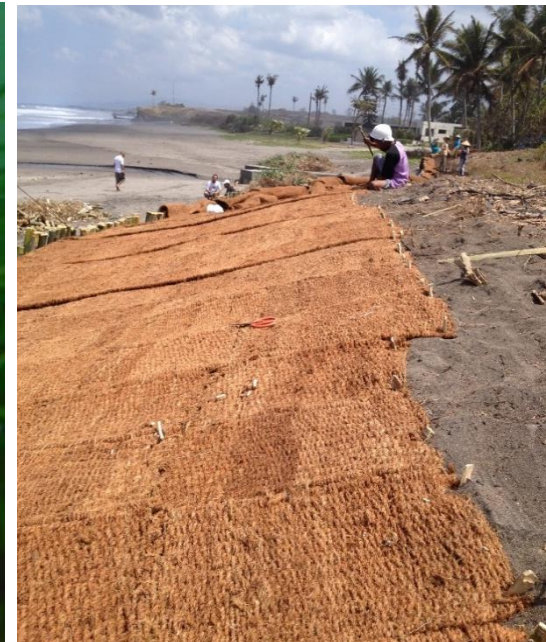
Coir fibre geotextile as filter, stabilization and initial shelter for a nature based revetement in Tabanan, Bali, Indonesien (David et al., 2016)
