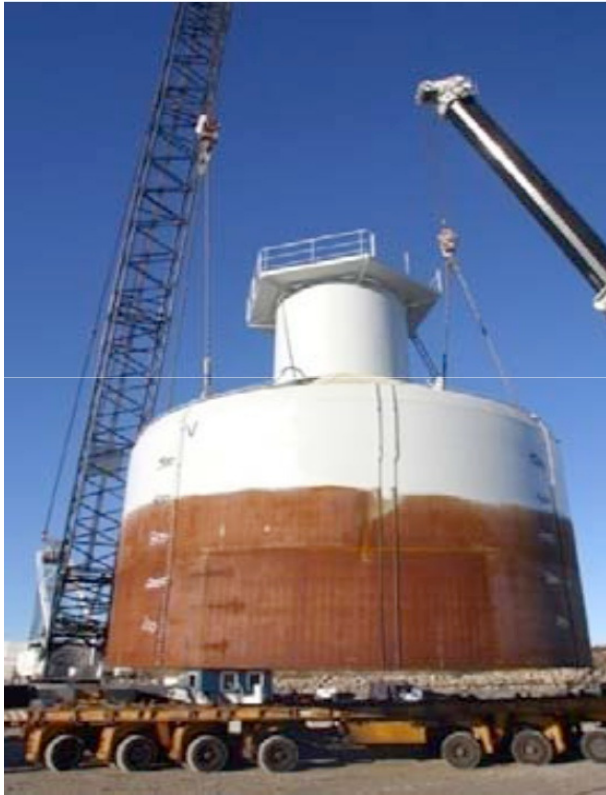
Bucket Prototyp in Fredrikshavn, Dänemark D = 12\text{ m} , L = 6\text{ m} (LeBlanc, 2009)
