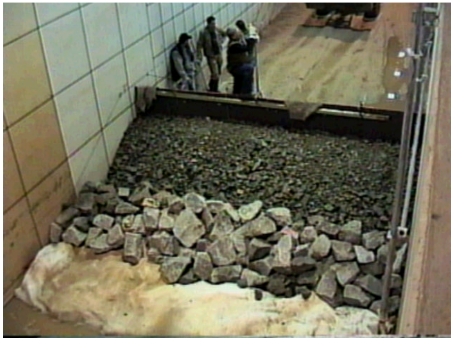
Fig. 8-3. Structure installation with an impermeable sheet in the middle
