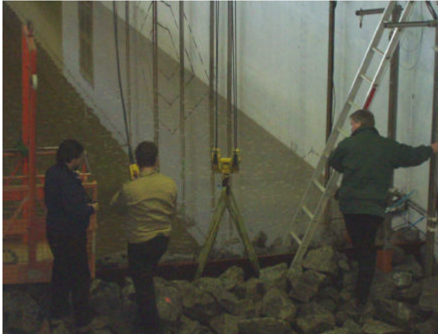
Fig. 8-4. Removal of impermeable sheet from middle of structure
