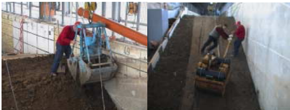
Fig. 6. Built in of Soil (left) and Compression of Soil in the Large Wave Flume (right)
