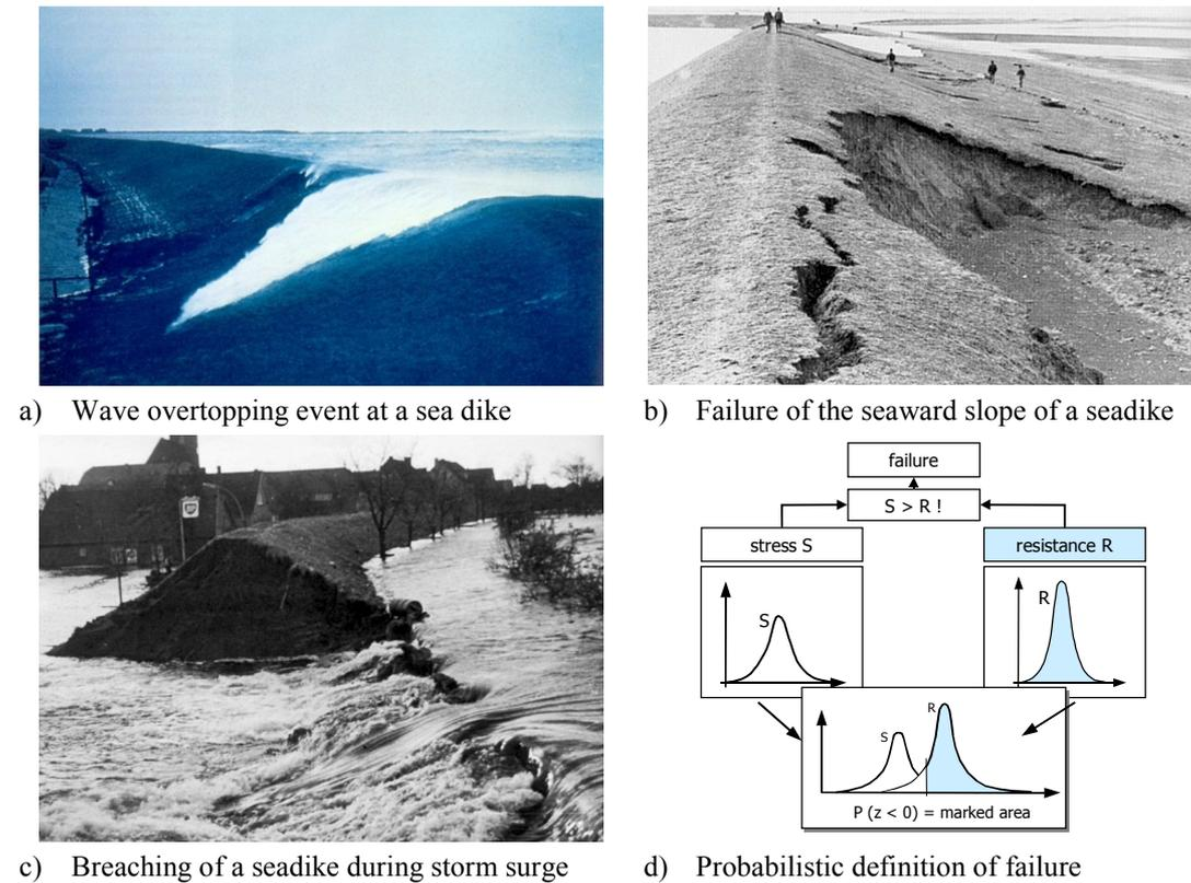
Fig. 3: Three example “failures” of a seadike
